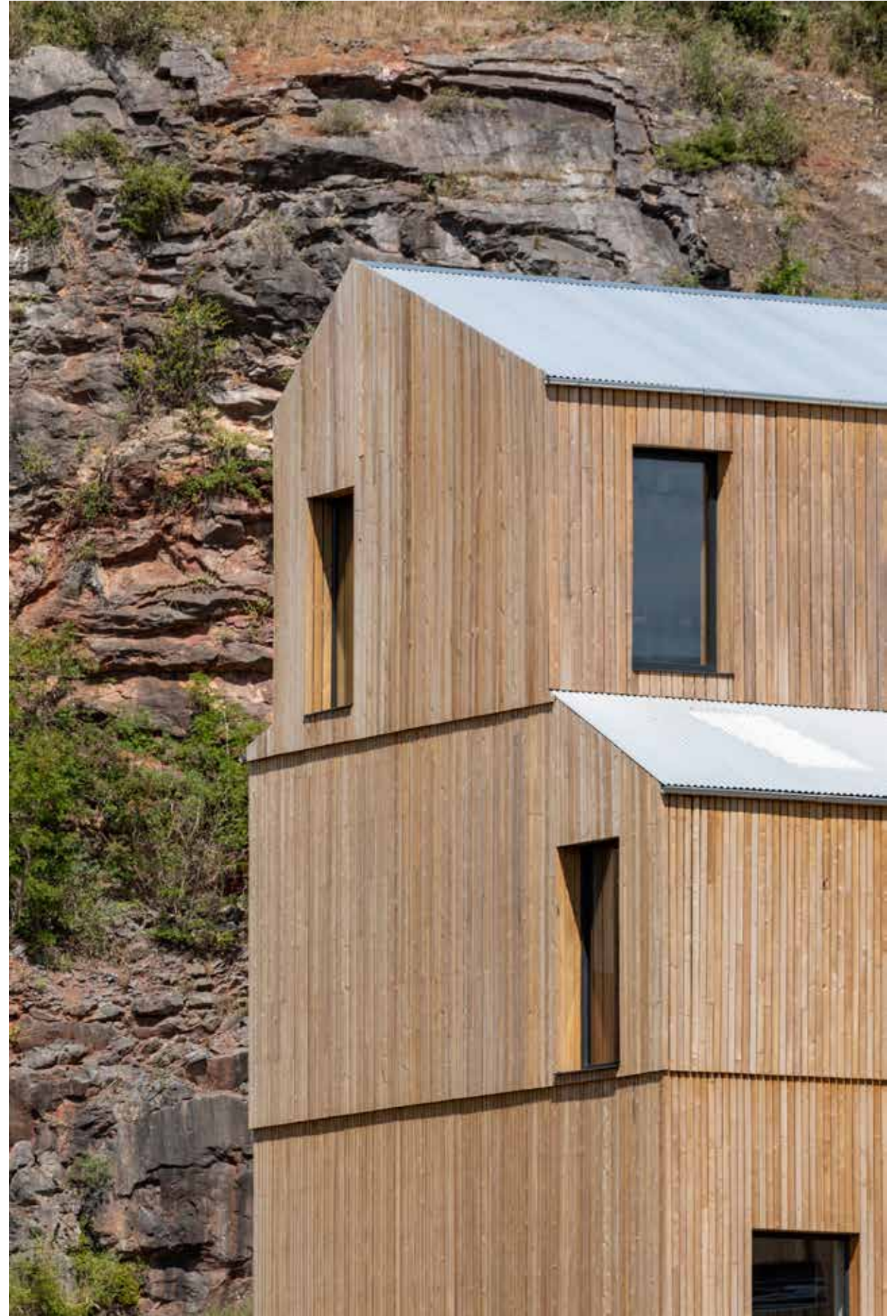
Charlie Bigham's West: Phase 1, Dulcote Quarry, Wells, Somerset Photo: Peter Cook
