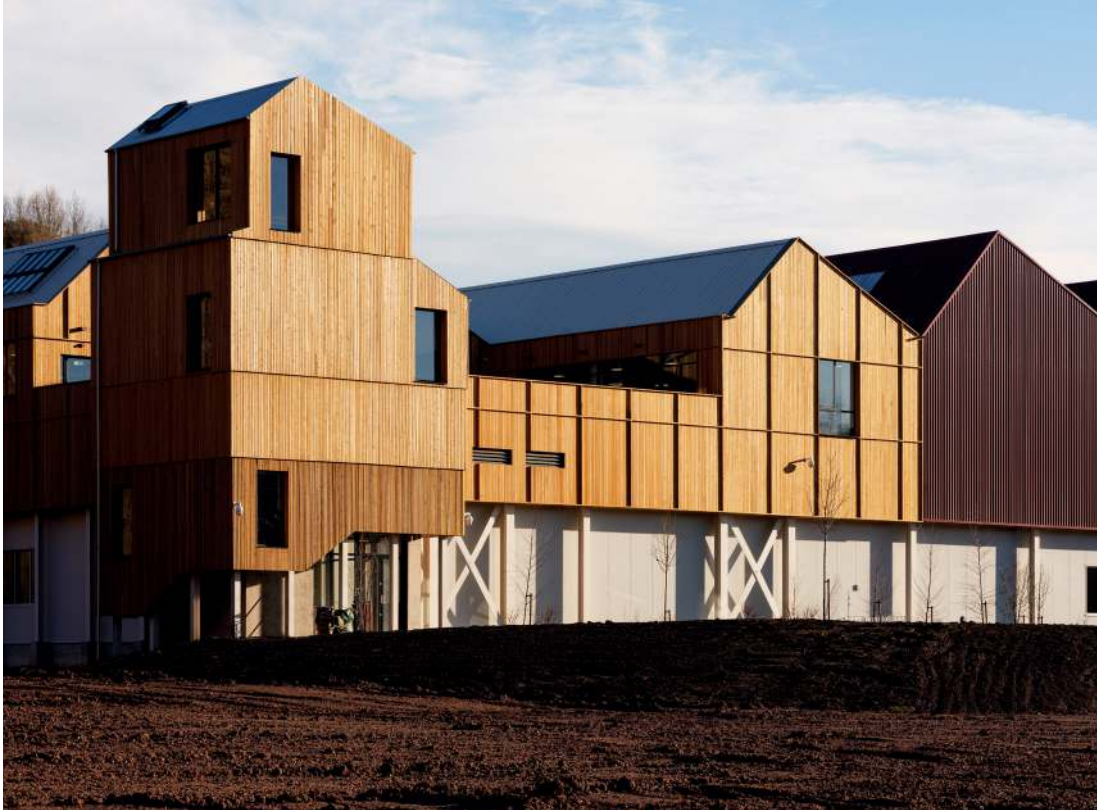
THE NEW CHARLIE BIGHAM'S WEST PRODUCTION FACILITY IS LOCATED IN A FORMER LIMESTONE QUARRY IN SOMERSET. UNUSUALLY FOR SUCH A BUILDING, ALL STAFF USE THE SAME ENTRANCE, SITUATED AT THE FOOT OF A TIMBER-CLAD TOWER
